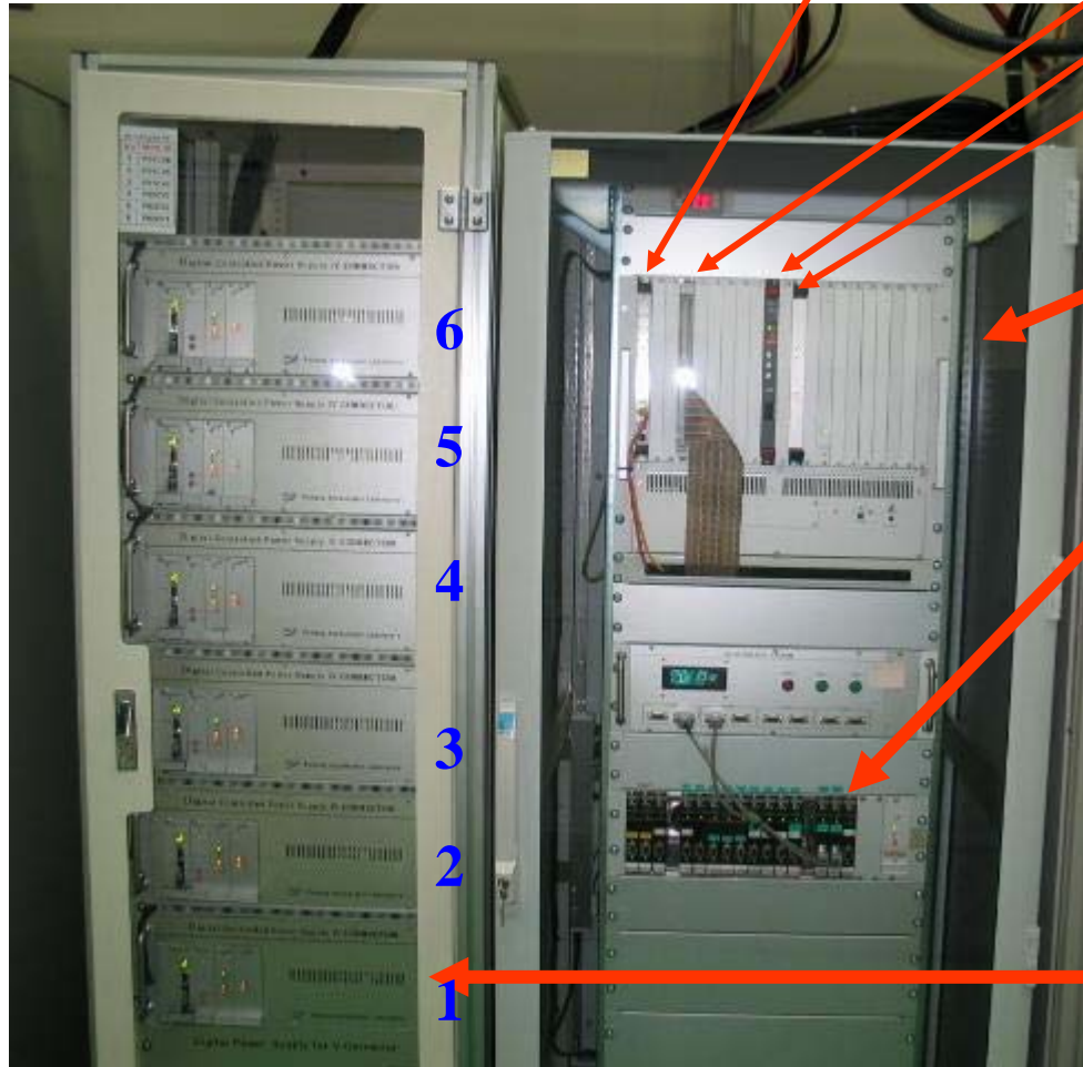
Digital PS and Control Rack
